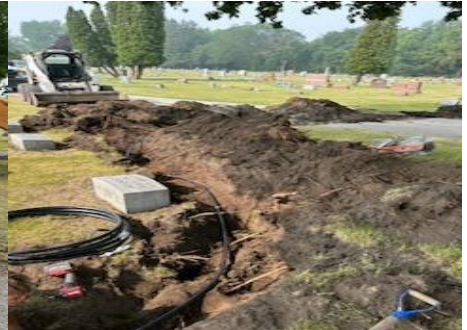
WATER LINE REPAIRS
